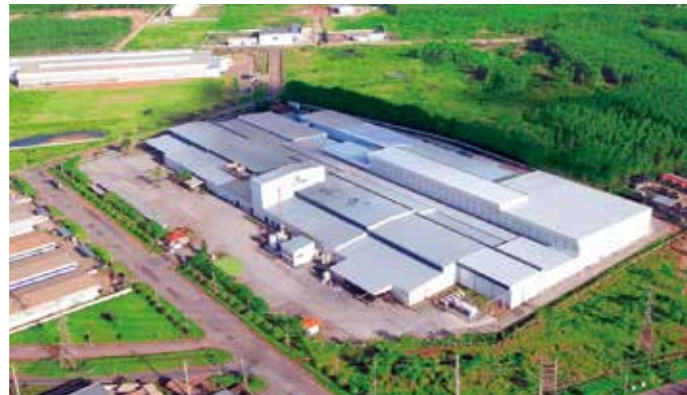
Oji Paper (Thailand)・Oji Label (Thailand) 工場全景
