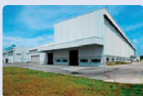
PT. PK Manufacturing Indonesia
