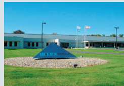
HI-LEX CONTROLS INC. LITCHFIELD PLANT (U.S.A.)
