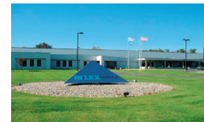
HI-LEX CONTROLS INC. LITCHFIELD PLANT (U.S.A.)
