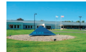
HI-LEX CONTROLS INC. LITCHFIELD PLANT (U.S.A.)
