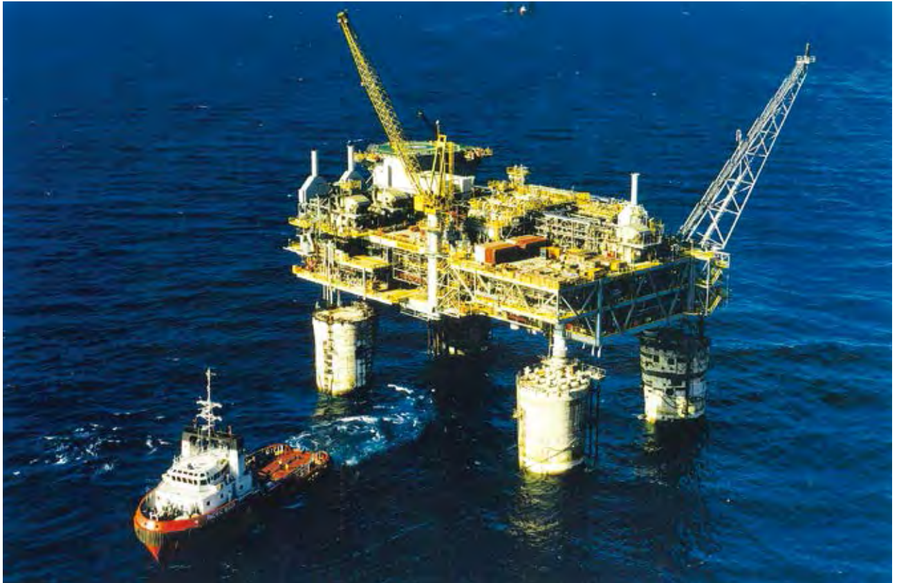
Wandoo B topsides and CGS undergoing commissioning after installation in early 1997
