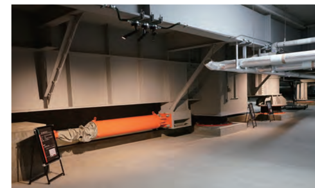
Seismic isolation equipment in Planet Saitama
